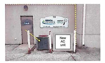
Note: The copper lines for the old AC unit are buried underneath the pavement. To reduce the cost, the new AC unit will be moved to the south and the new lines will be installed on the outside of the building. The lines will be covered and run up the corner of the building and along the top above the door light. At a later date, City Staff will paint the copper line shield.
